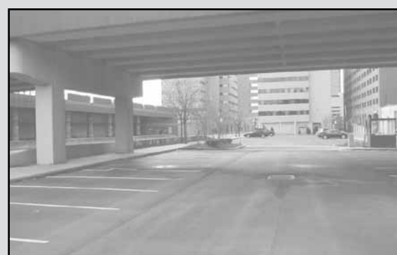
Underneath the MLK overpass. This section must be addressed in all design submissions. Photo by Danny Mayer.
