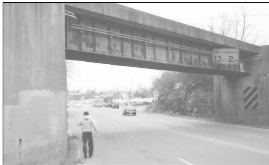
This is not a safe pedestrian thoroughway.
