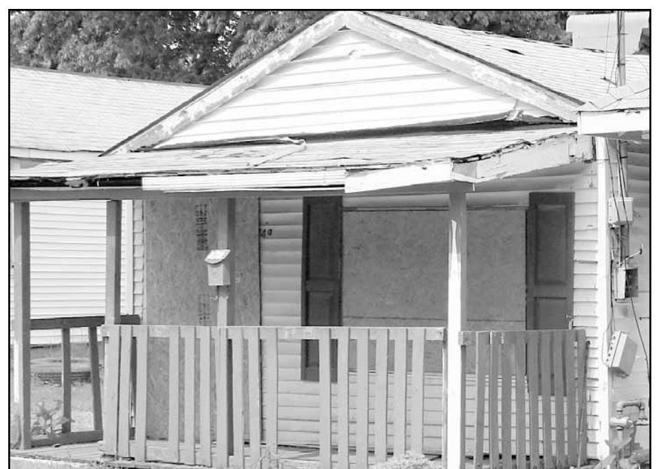
Plywood boards cover the windows of this Lexington property. Photo: Lisa Schroot.
